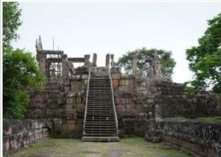
>> (From left): along with buttress facing north; western face.
