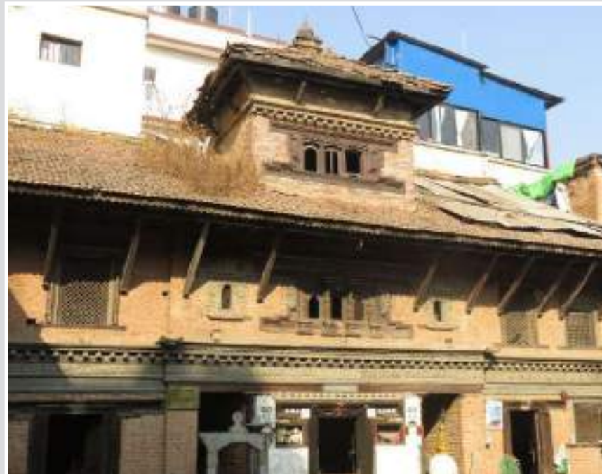
« Napichandra Mahavihara popularly known as Duntu Bahi is located to the north of Patan Durbar Square, UNESCO World Heritage zone of the Kathmandu Valley. The original shrine building suffered extensive damage after the 1934 earthquake and was rebuilt in 1980's.
