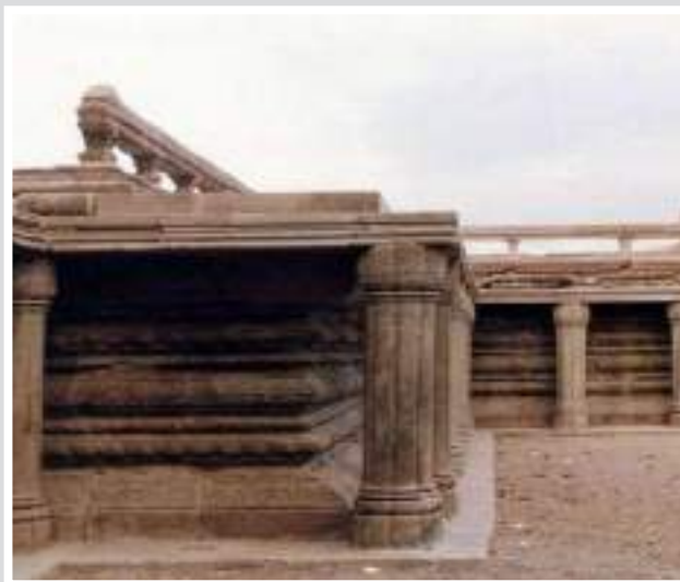
(From Top): North West corner of Ranga Mancha (Before Conservation); North West corner of Ranga Mancha (After Conservation)
